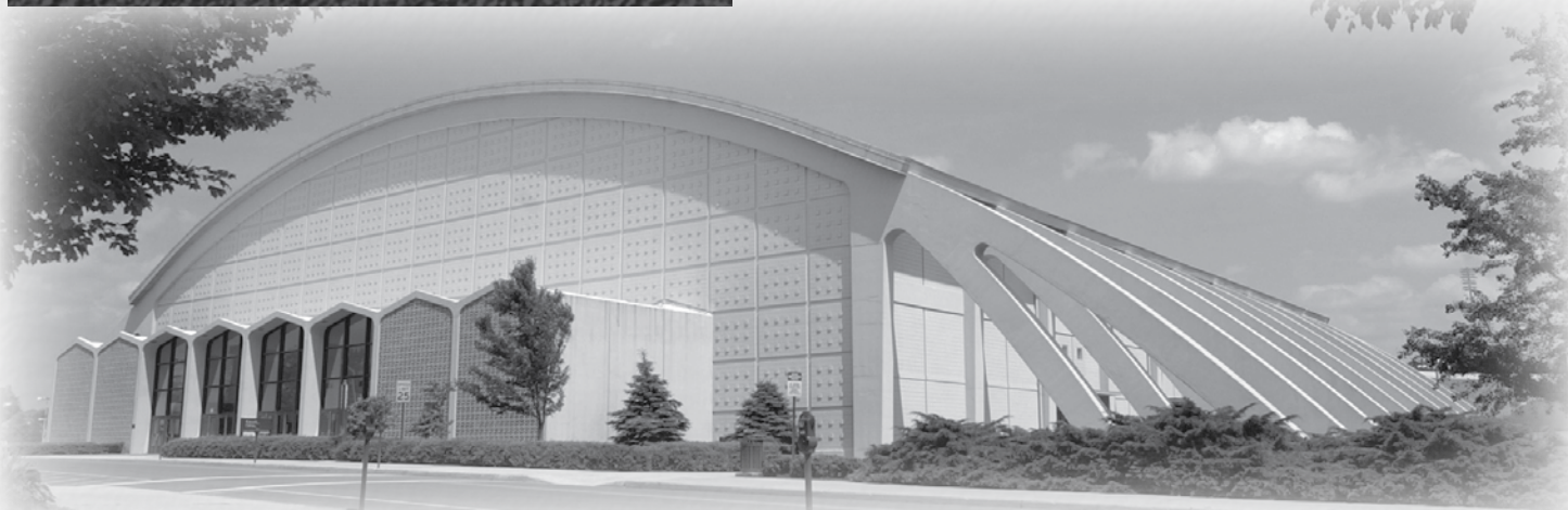
Cassell Coliseum, home of Hokie wrestling, is easily identified among all other buildings on campus.
