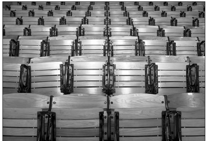
Newly-refinished seats were only the first stage in major renovations that are being completed in Cassell Coliseum this fall.
