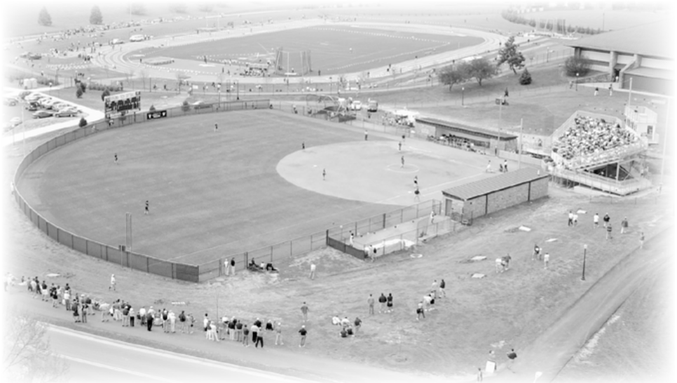
With permanent seat-back bleachers, handicap accessibility and a modern press box, Tech Softball Park has become one of the best facilities around and always draws great crowds to Hokie softball games (left).
