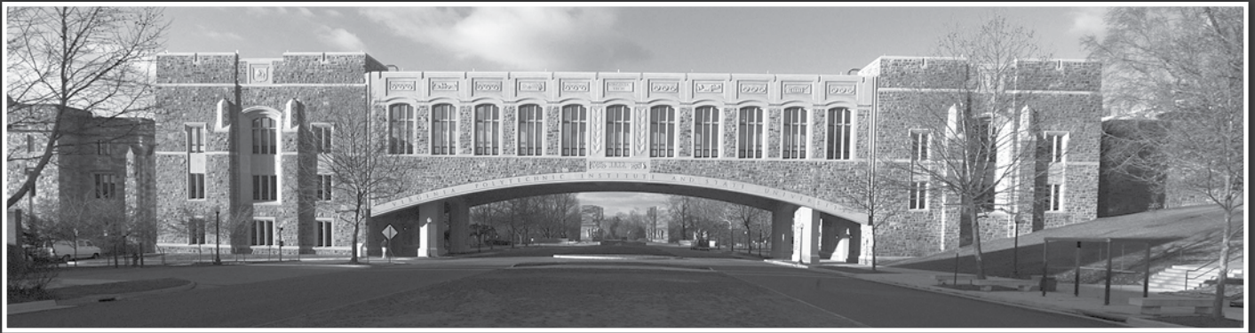
Torgersen Hall, home to Virginia Tech's Advanced Communications and Information Technology Center, provides a high-tech environment in which researchers, teachers and students can interact in innovative and effective ways. The building includes high-tech auditoriums, observational booths for watching and taping experimental teaching techniques, the CAVE – Tech's sophisticated virtual reality environment for advanced research and learning, and an electronic reading room occupying the arch that spans Alumni Mall.
