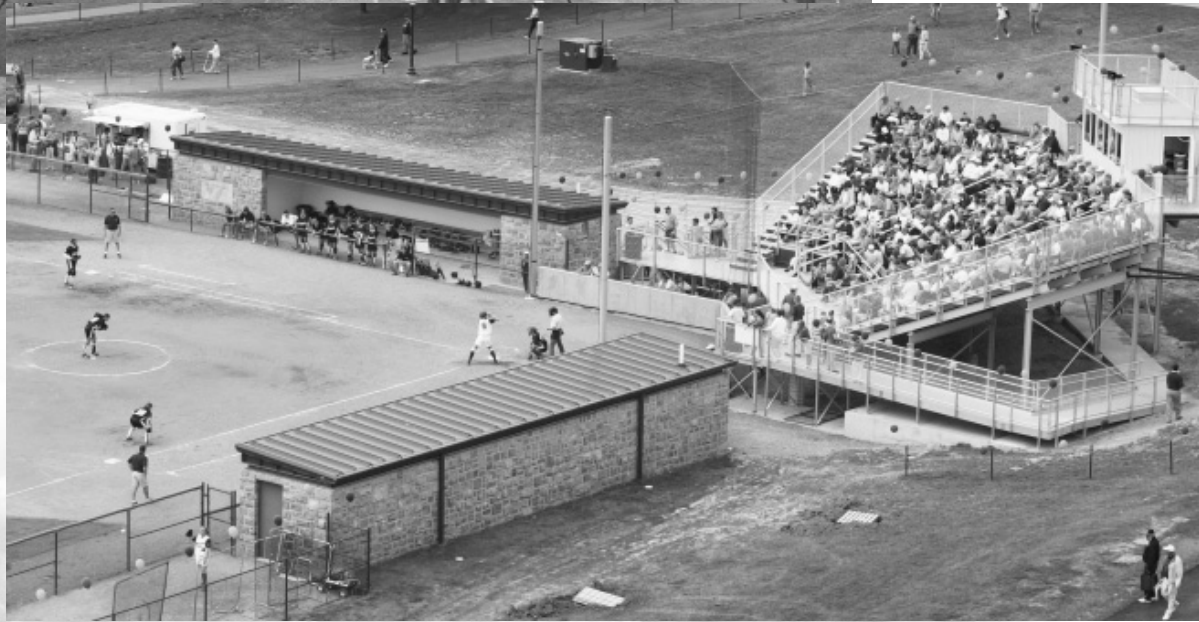
Tech's relatively-young softball program has only been in existence for eight years, but — like many Tech athletic teams — it has already built a reputation for winning. New bleachers and a press box have been added to their facility over the last few years.
