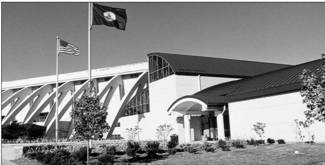
The Merryman Center is one of the most unique buildings on the beautiful Virginia Tech campus.
